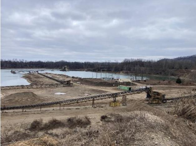
South view of pit showing conveyor route from dredge to screen shaker feed to jaw crusher (STOP 2)
